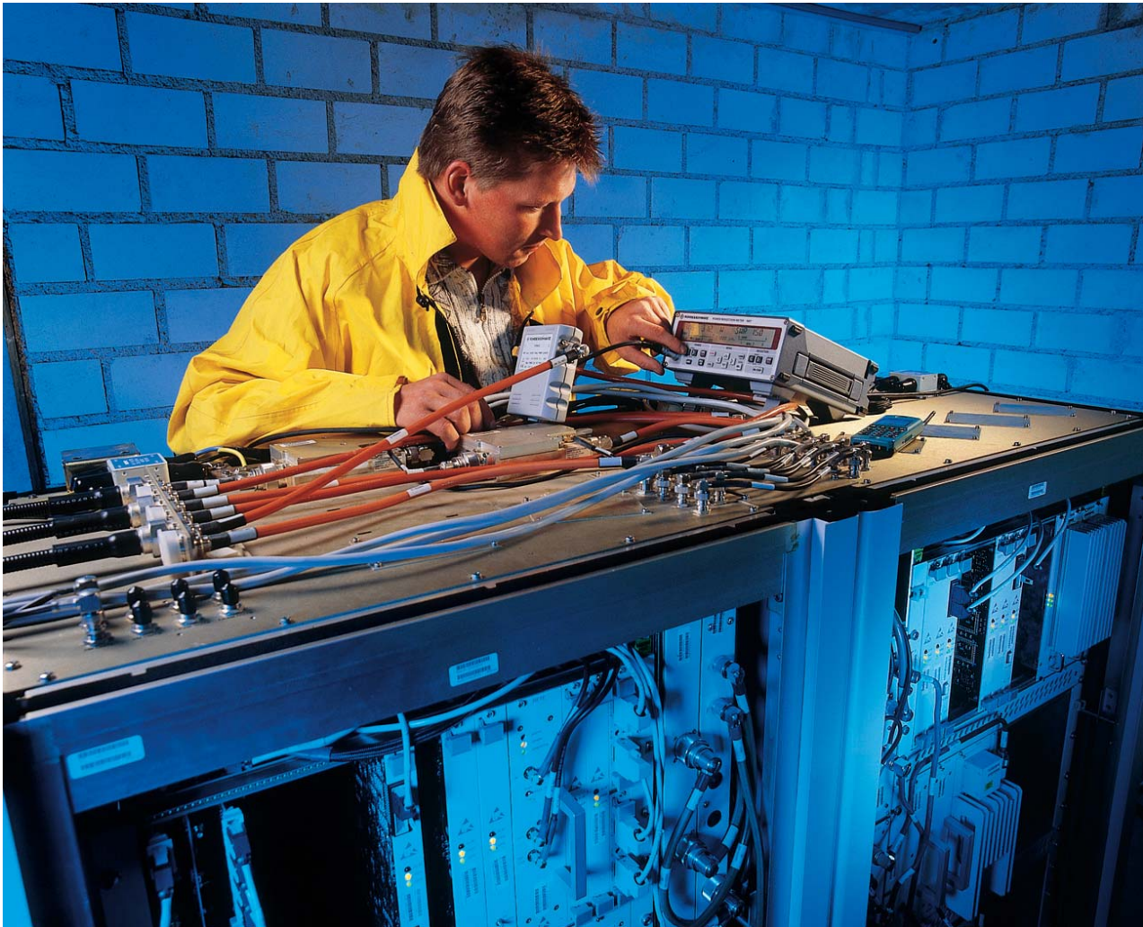
Installing a mobile radio base station with R&S R&S NRT (photo 42667)
